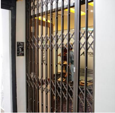
Fully framed with a neat and compact sash, galvanised steel trellis-patterned security barriers are ideal for doors, windows and other openings.
